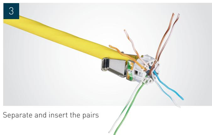
Separate and insert the pairs
